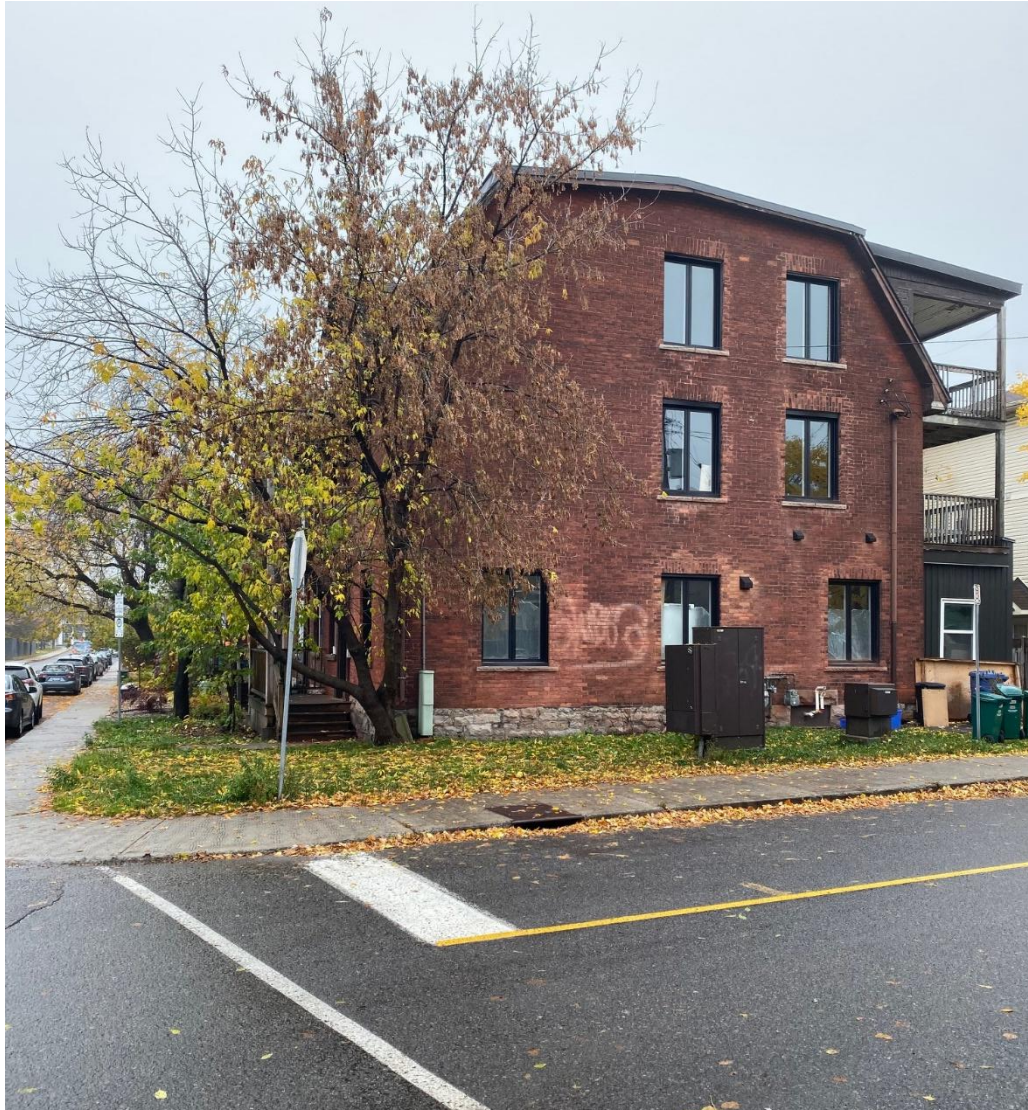
The mural would be installed on the graffiti-impacted north facing wall
