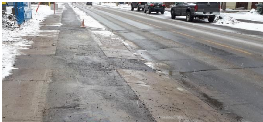
Figure 1 - Road Cut for Development Servicing
