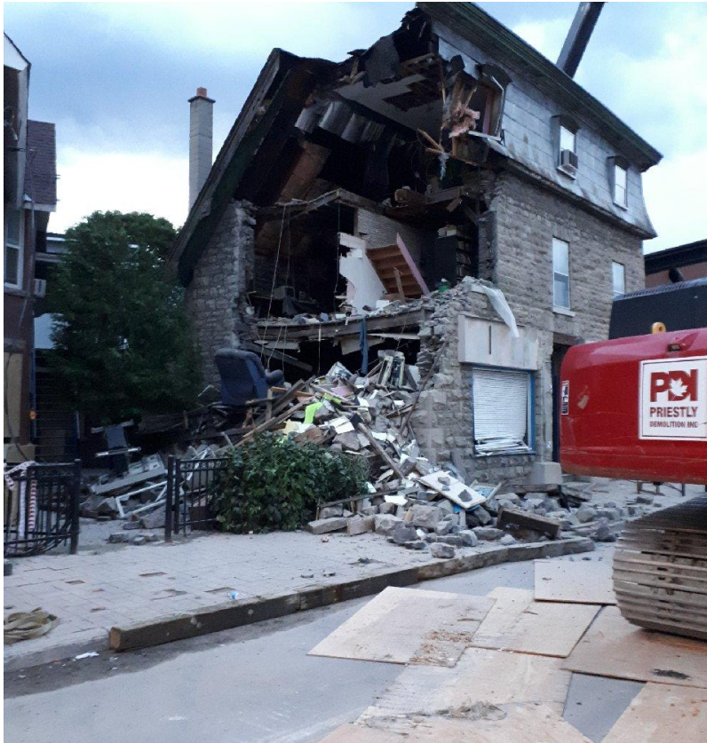
1119 Wellington Street West following partial demolition
