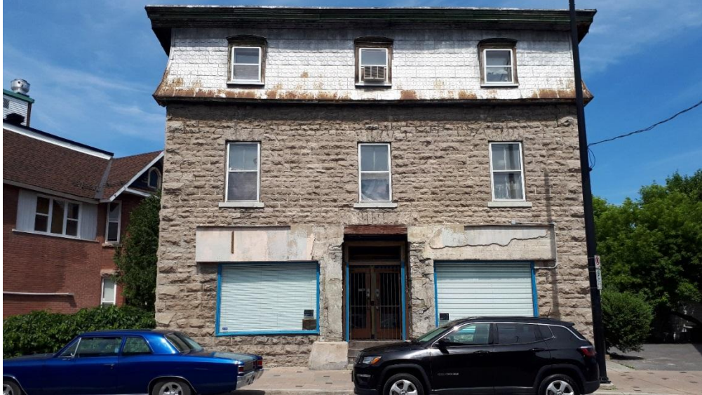
1119 Wellington Street West prior to collapse
