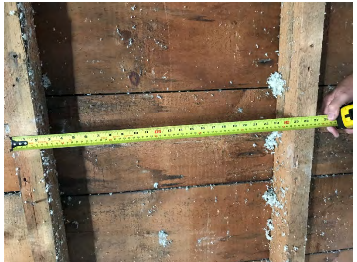
Studs Picture 2 – Spacing of existing East Wall
