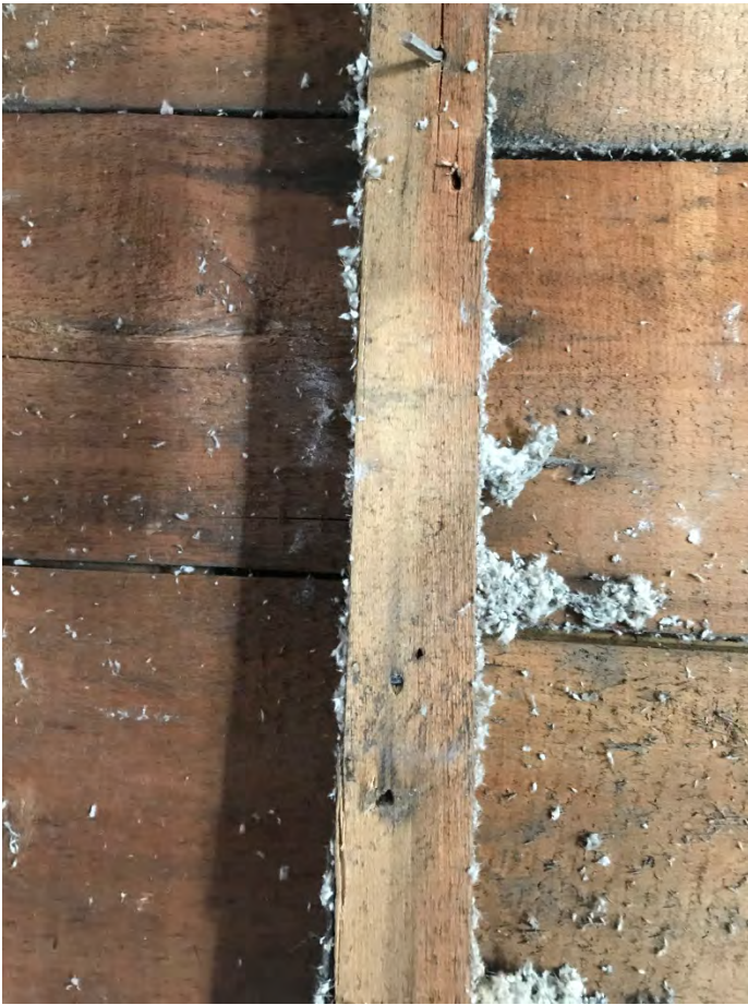
Picture 3 – East Wall Stud
