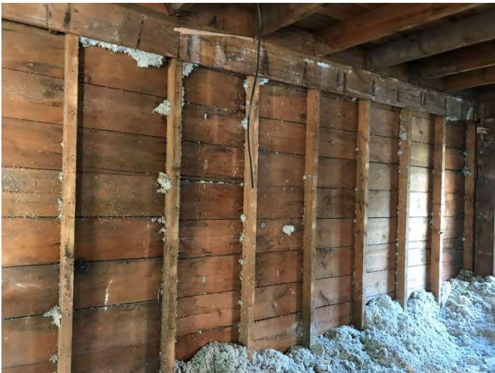
Existing Picture 1 – Existing East Wall
