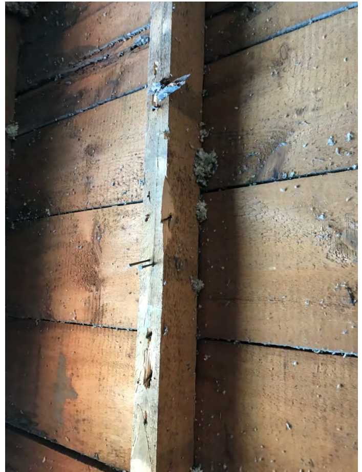
Picture 4 – East Wall Stud
