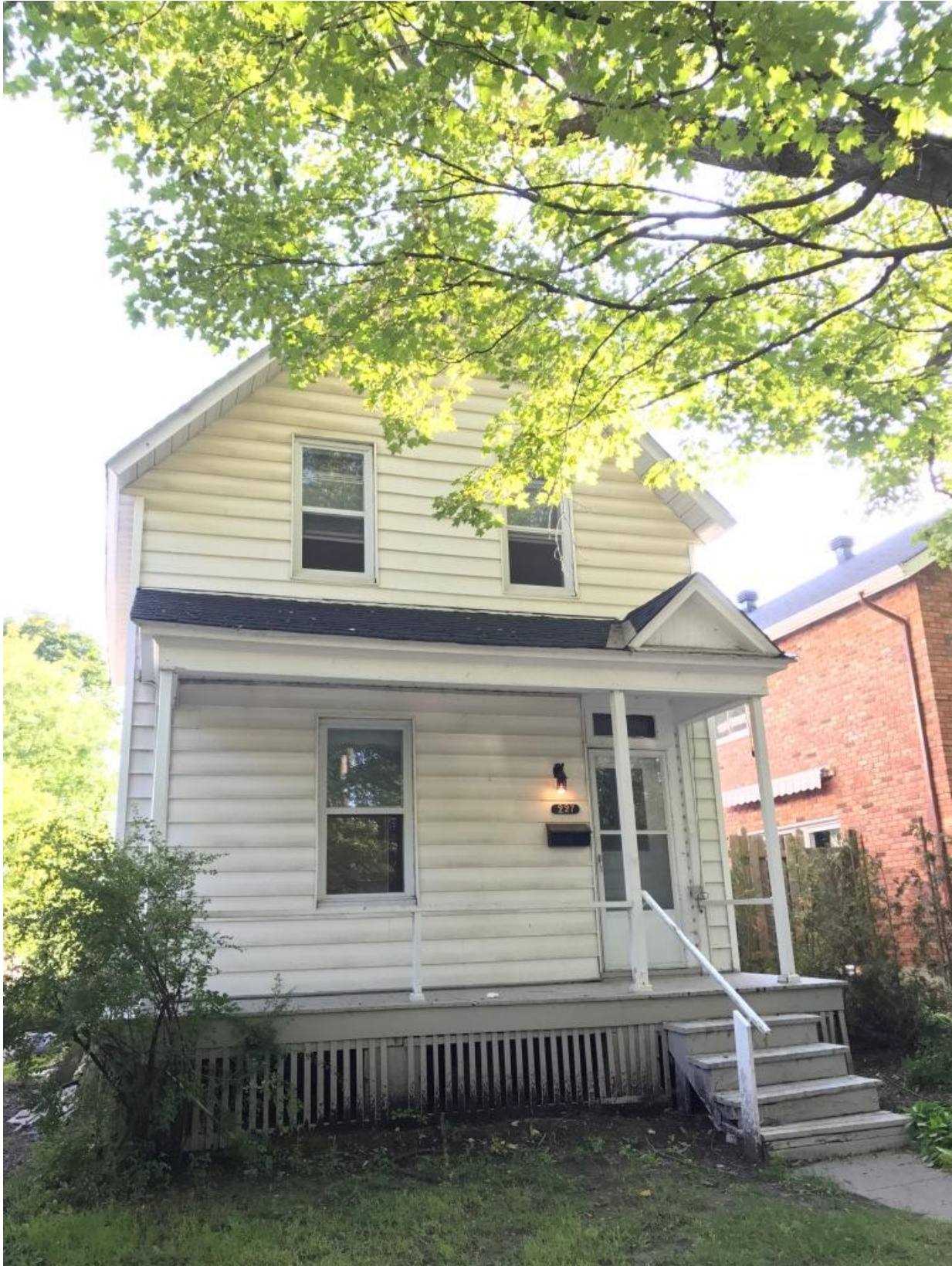
Document 2 – Front façade, former building, 227 MacKay Street
