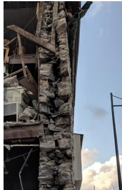
Figure 3: South Elevation - Empty Wall Core
