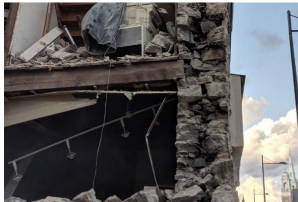
Figure 1: Bearing of 2nd Floor Joist
