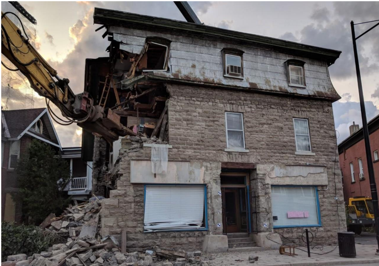
Figure 2: Extent of Partial Demolition (approx.)
