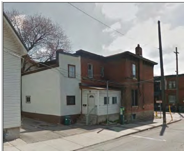
Figure 4: 423-425 McLeod Street, side (west) and back (north) façades of existing multi-unit residence. (Google)
