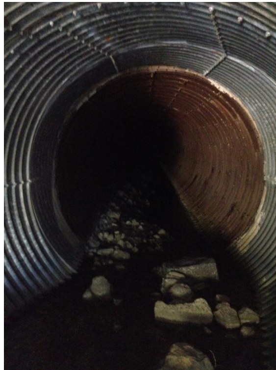
Figure 3.2 Transition from CSP to Liner Plate – July 2012
