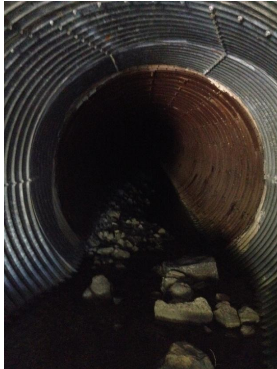
Photo Courtesy of KWH Pipe
